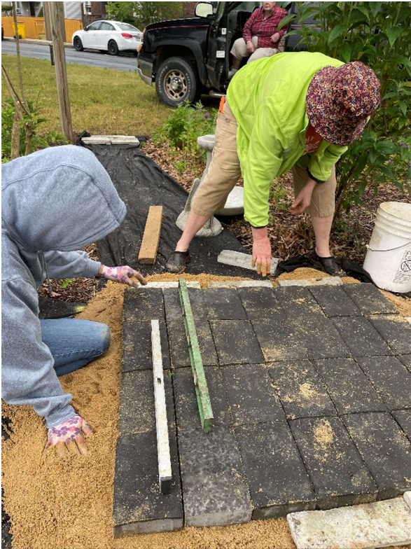
Regina and Jane laying block
